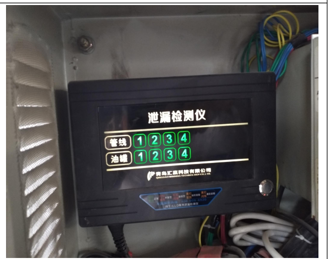
输油管线渗漏检测
